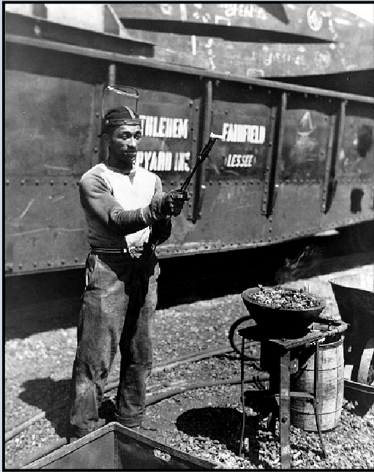
Smith, Roger, photographer. Baltimore, Maryland. A rivet heater preparing to toss a red hot rivet to be used in the building of the Liberty ship SS Frederick Douglass at the Bethlehem-Fairfield shipyards. May. Photograph. Retrieved from the Library of Congress, < www.loc.gov/item/2017851658/ >.
